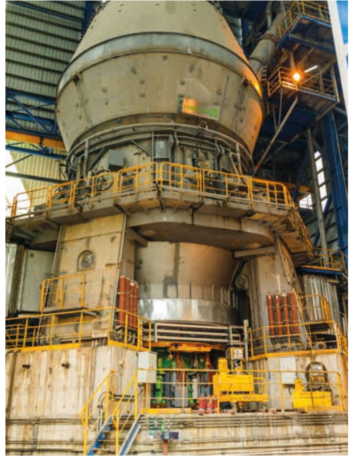
Mfamosing Vertical Cement Mill
