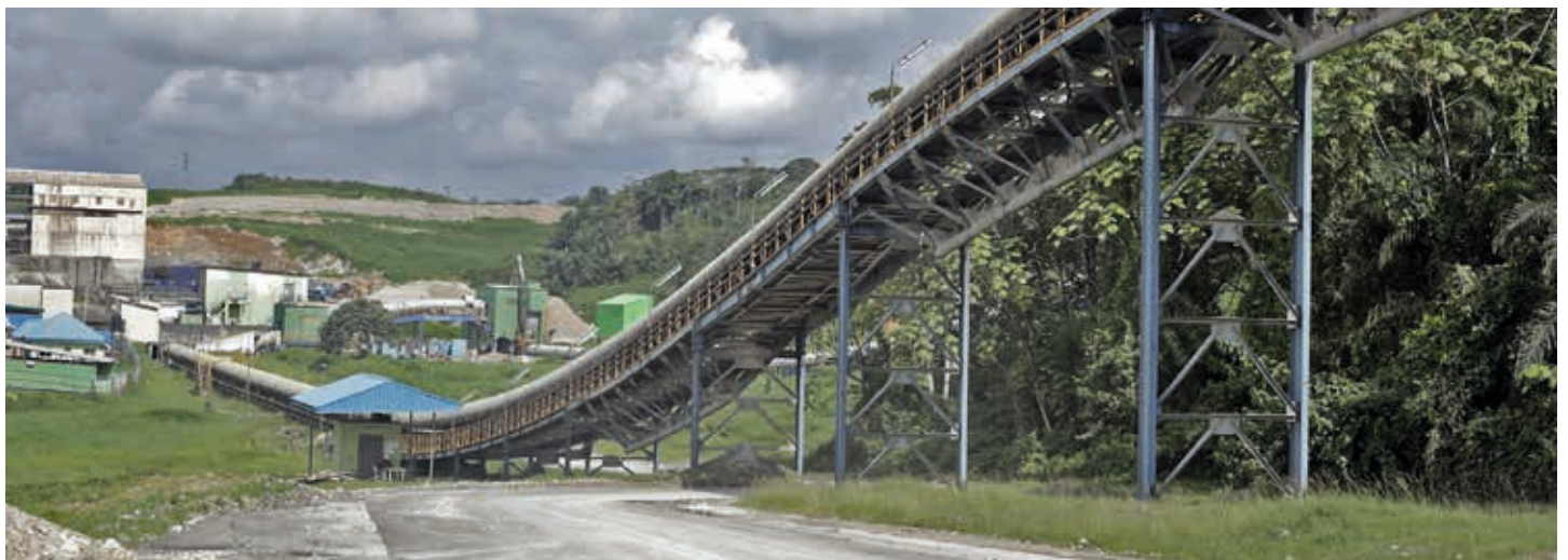
Conveyor Line, Mfamosing Plant
