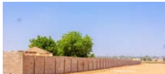
810-metre fence at Bajoga 2 Primary School
