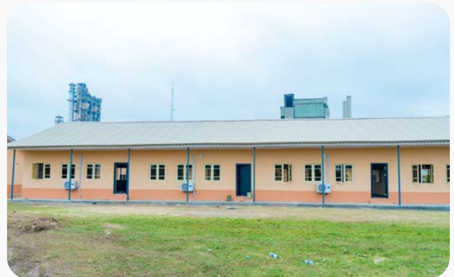
Remodeling of Christian Pelamourgues Primary School, Agbesi
