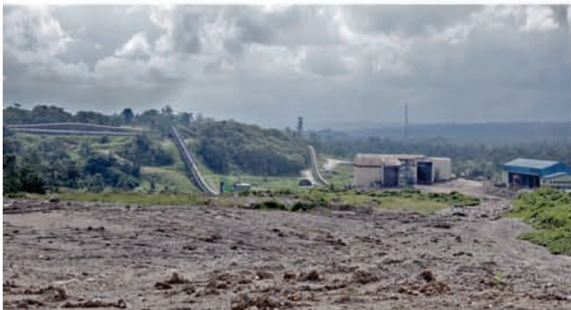
FIG B: Site preparation at the Mfamosing Quarry for reforestation
