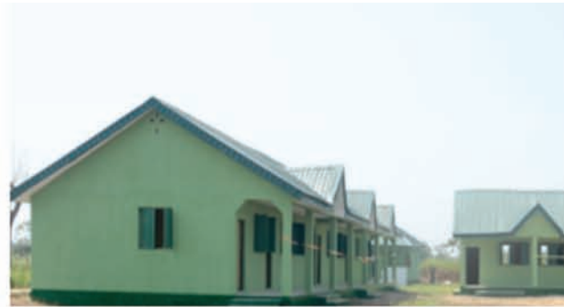
A newly constructed block of classrooms in Akinbo Community, Ogun state
