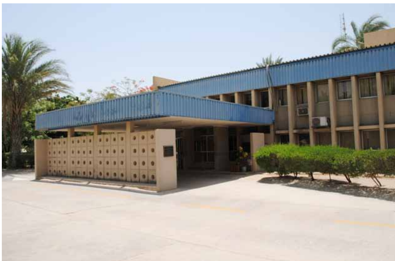
Ashaka Cement head office.
