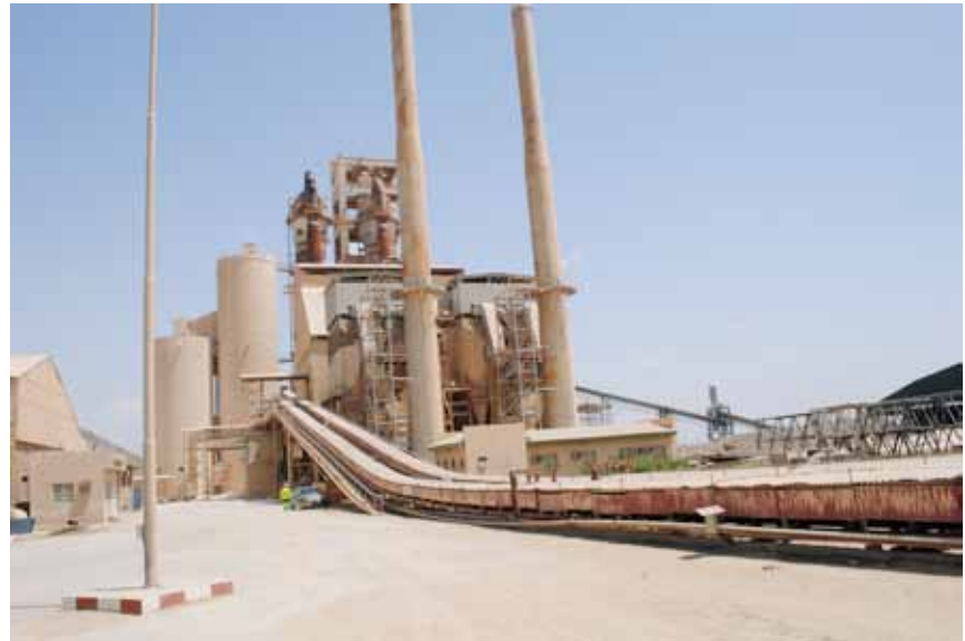
AshakaCem Plc cement plant.
