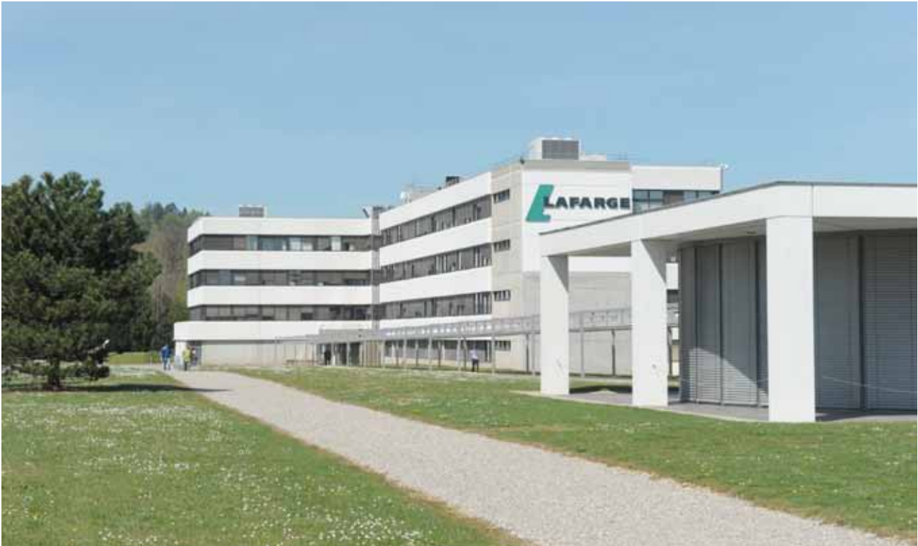
Lafarge Research Centre, Lyon.
