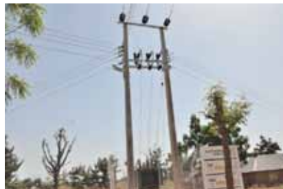
Lakwalak electrification project.
