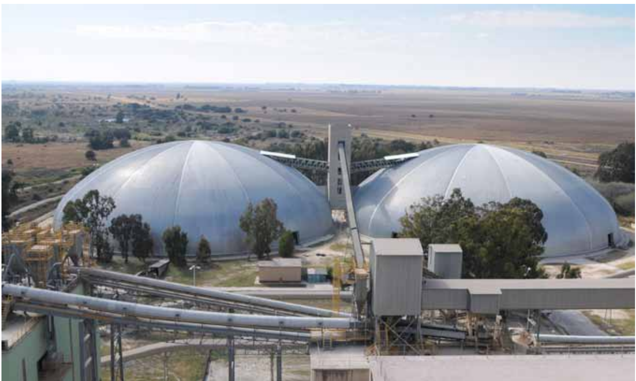
High angle view of Lichtenburg cement plant, South Africa.
