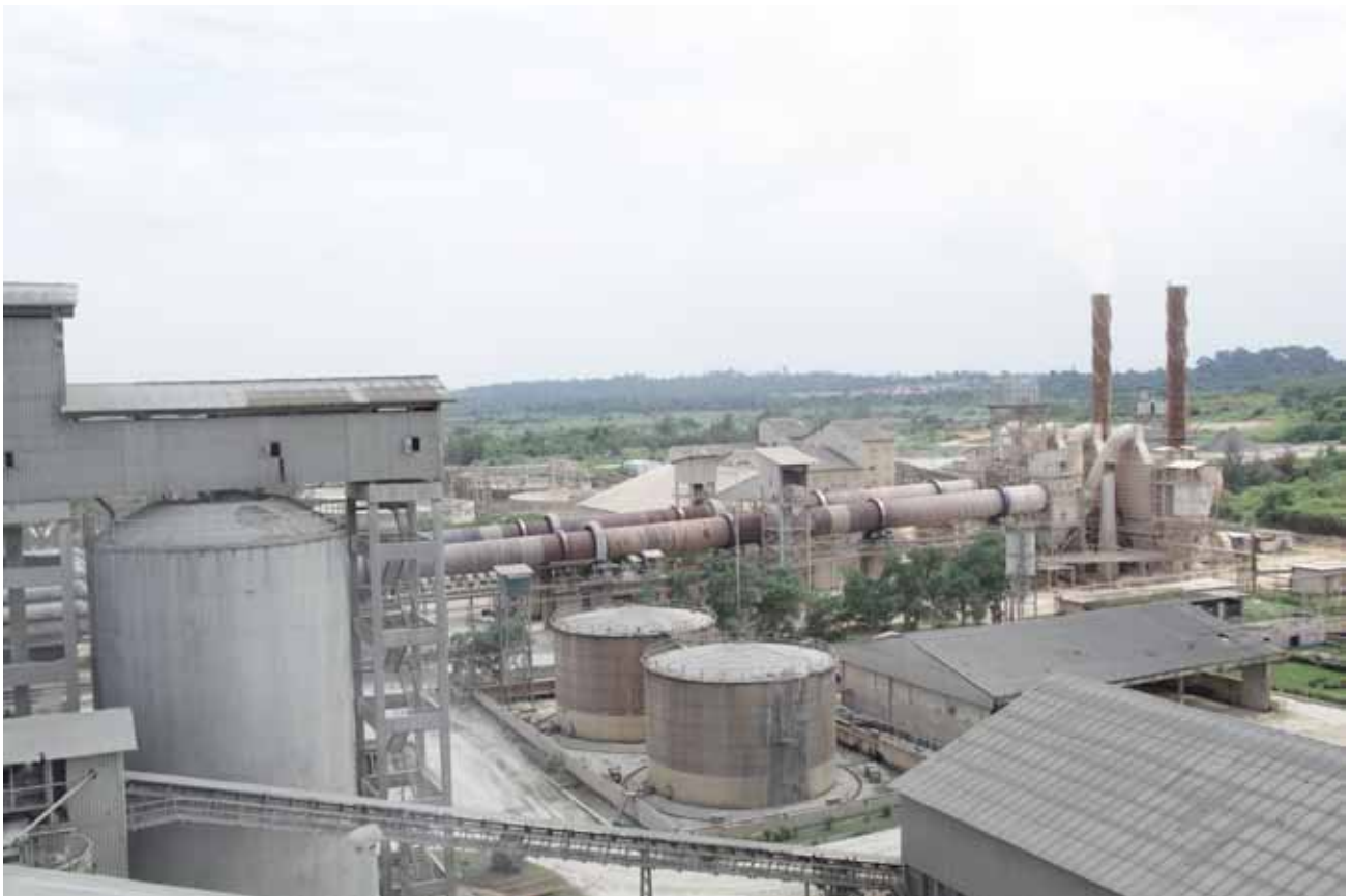
Aerial view of Sagamu Plant, WAPCO Operations.
